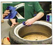
Both the rim and hub are cleaned thoroughly to remove any remaining glue that may prevent the replacement trim from seating properly
