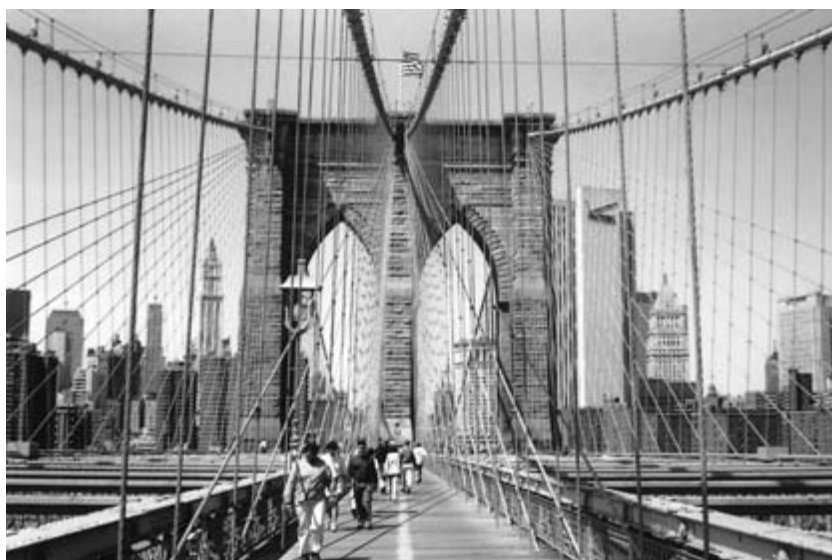
Fig. 3.15 Brooklyn Bridge, New York City.
