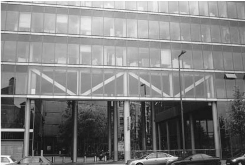
Fig. 12.5 Truss in façade, Sony Centre, Berlin.
