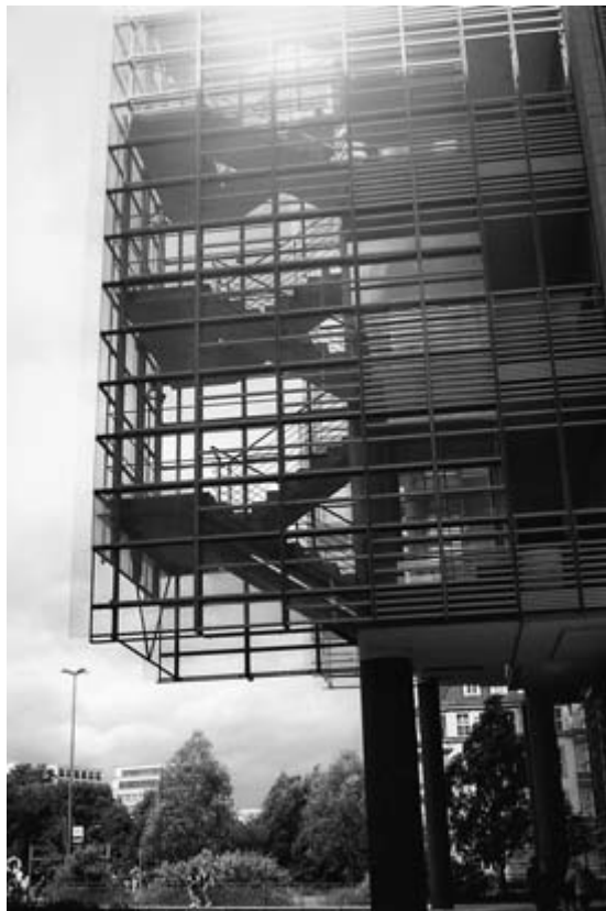
Fig. 1.3 A very visible staircase. How is it supported?
