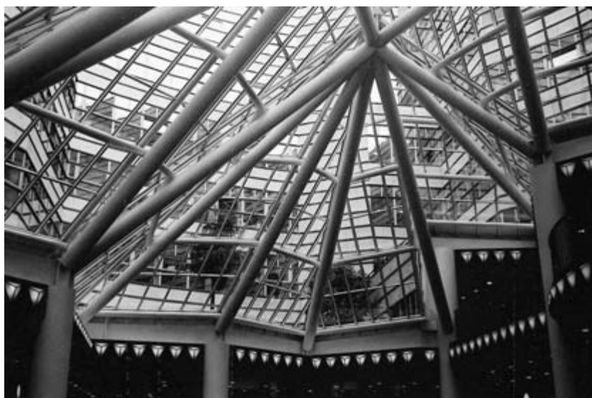
Fig. 1.2 Roof structure of Quartier 206 shopping mall, Berlin.
