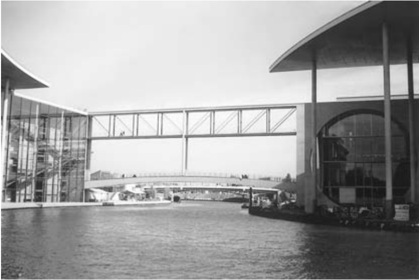
Fig. 12.4 Trussed bridge across River Spree, Berlin.
