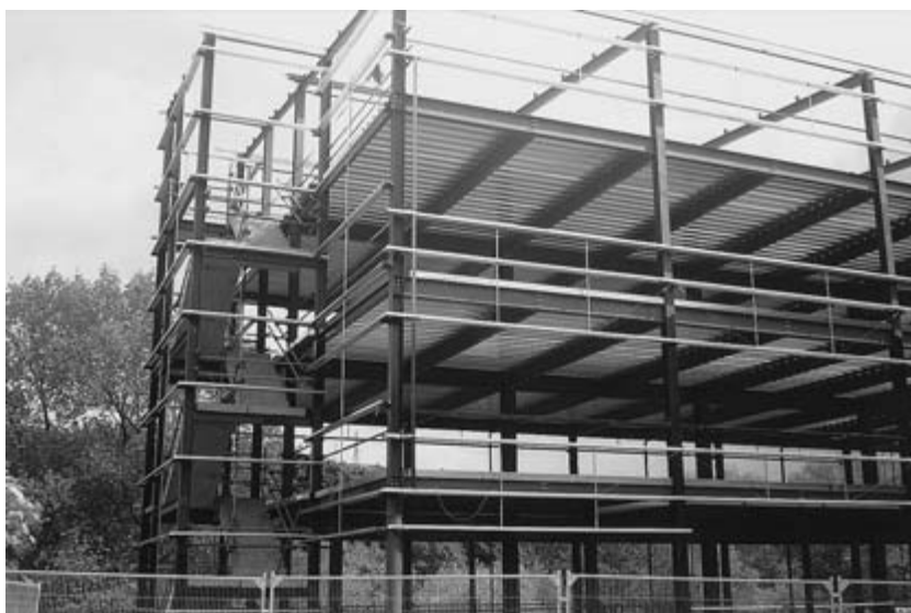
Fig. 22.1 Steel-framed office building under construction.
