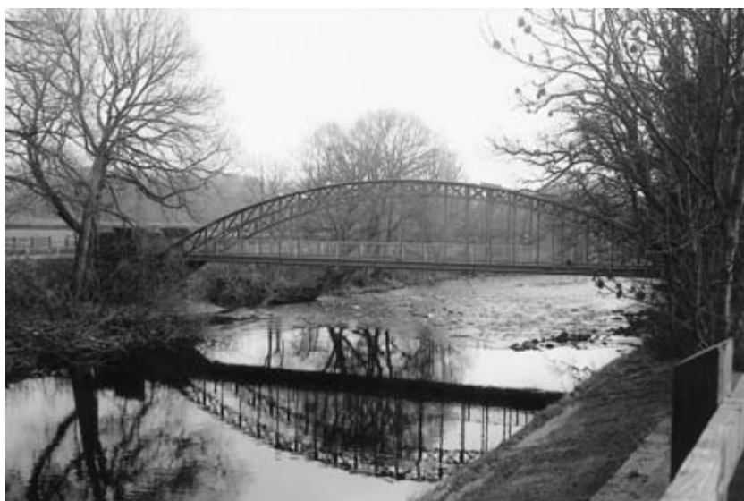
Fig. 6.1 Steel arch bridge.
