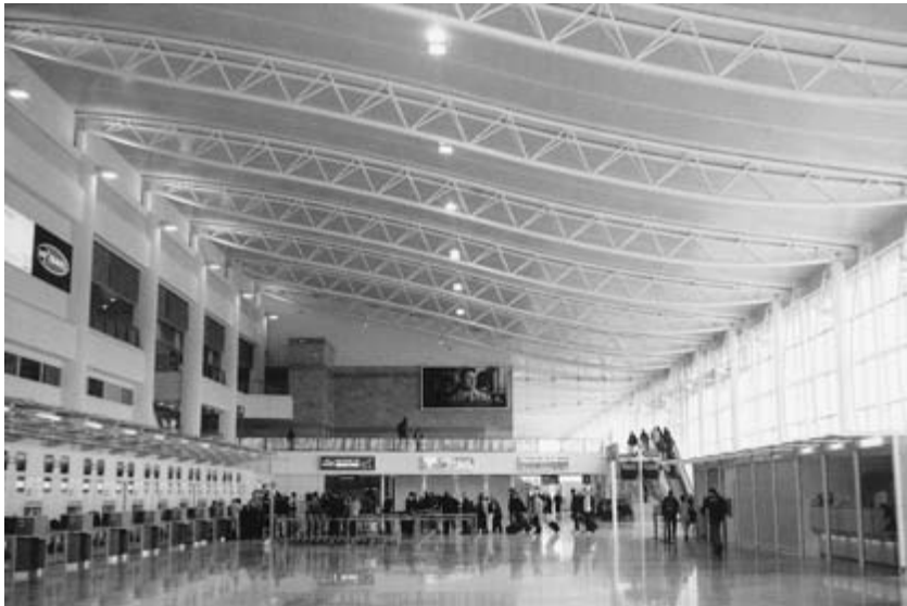
Fig. 23.7 Triangular lattice trusses supporting terminal roof, Liverpool John Lennon Airport.
