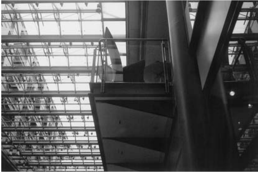
Fig. 16.25 Cantilevered balcony in shopping centre.
