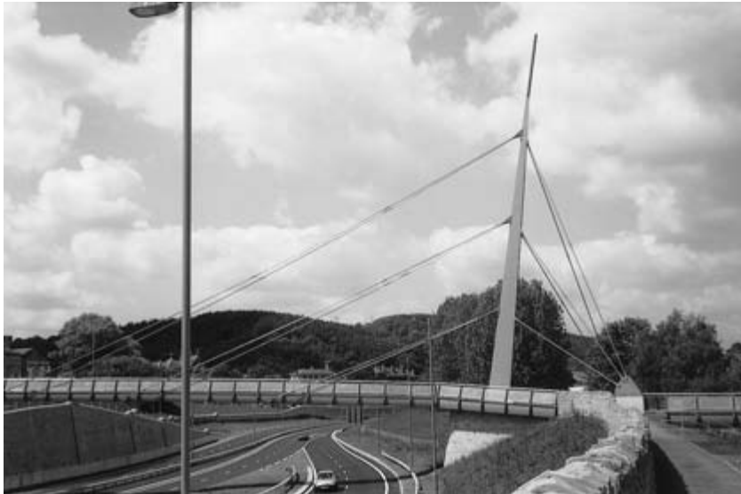
Fig. 17.3 Cable-stayed bridge, Bingley bypass, West Yorkshire.
