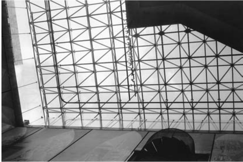
Fig. 15.7 Steel space frame roof, Lille Europe metro station, France.
