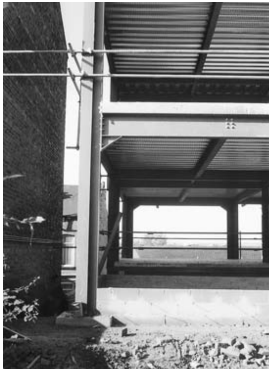
Fig. 9.2 Steel-framed building under construction.
