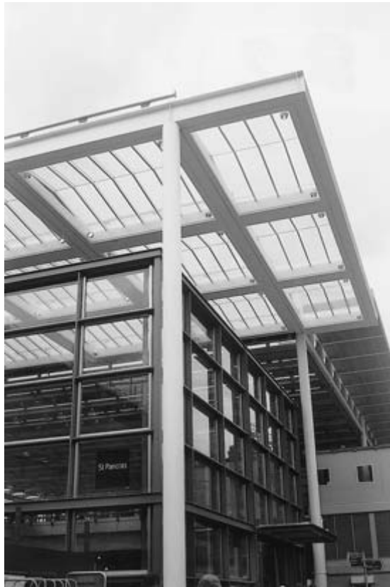
Fig. 10.8 St Pancras 'interim' railway station, London.
